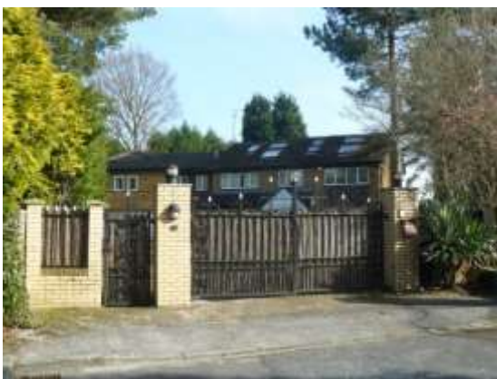
Photograph 19: Brick Piers with Metal Gates, Blenheim Road
