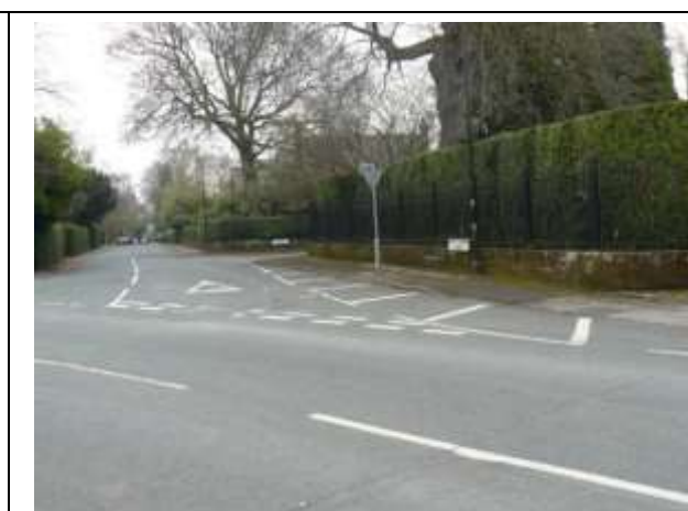
Photograph 28: Inappropriate Road Markings
