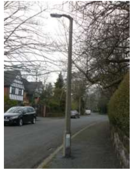
Photograph 30: Concrete Lamp Post
