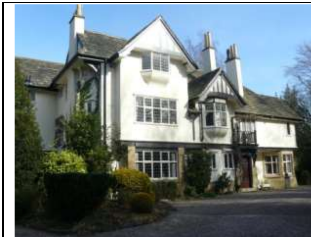
Photograph 5: Brick Property, Half Rendered, Black and White Timber Detailing
