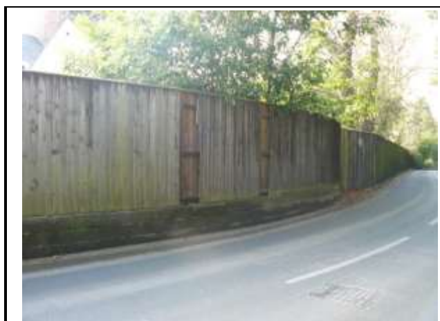
Photograph 25: Timber Panelled Fence
