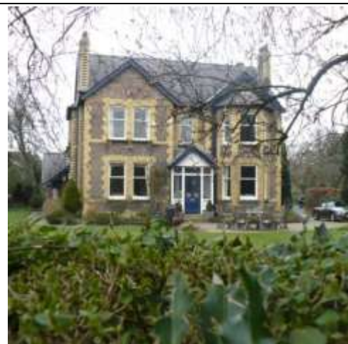
Photograph 6: Victorian Property with Polychromatic Brick Detailing
