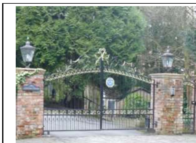
Photograph 27: Modern Gates and Gate Piers
