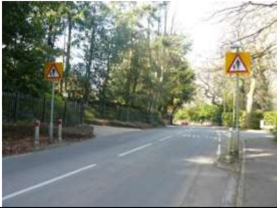
Photograph 15 : Signage Along South Downs Road
